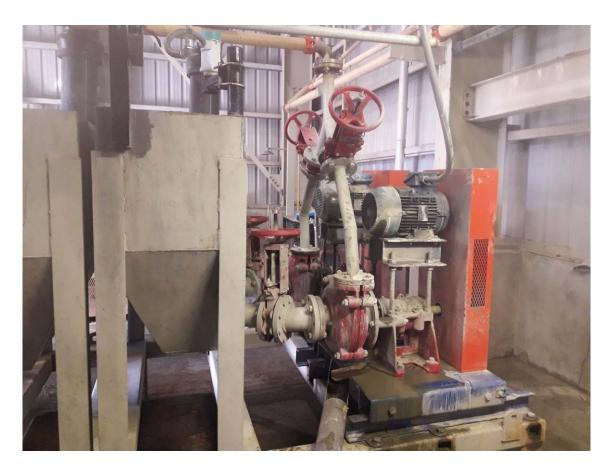
A major mining company dedicated to gold and silver extraction had two vertical pumps for repumping mining pulp into a flotation cell.
